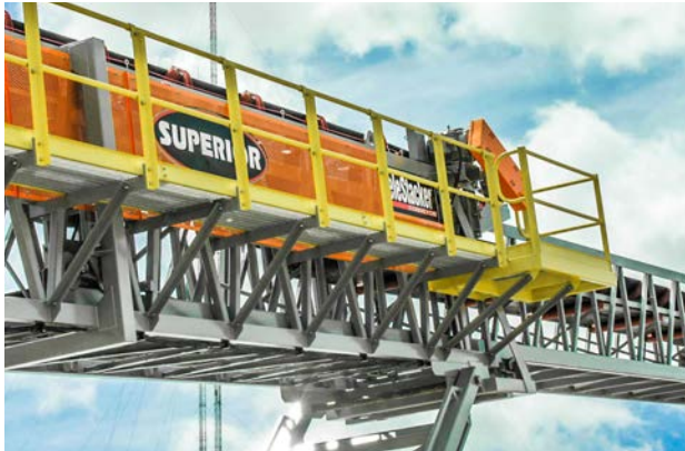
WALKWAY (ON MAIN CONVEYOR)
