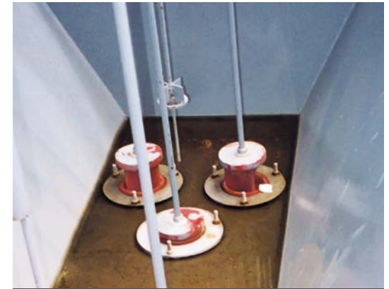
URETHANE DISCHARGE VALVES
