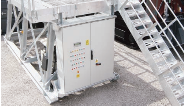
Complete Cone Starter Panel
