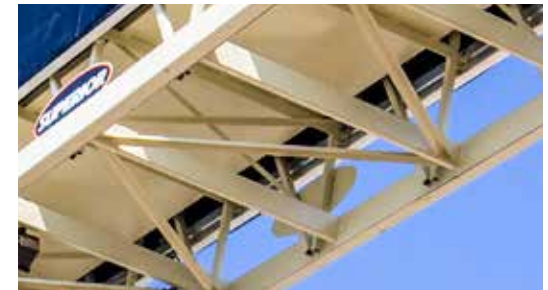
C/ STINGER CROSS BRACING
