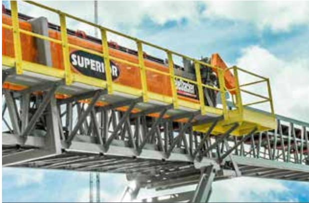
WALKWAY (ON MAIN CONVEYOR)
