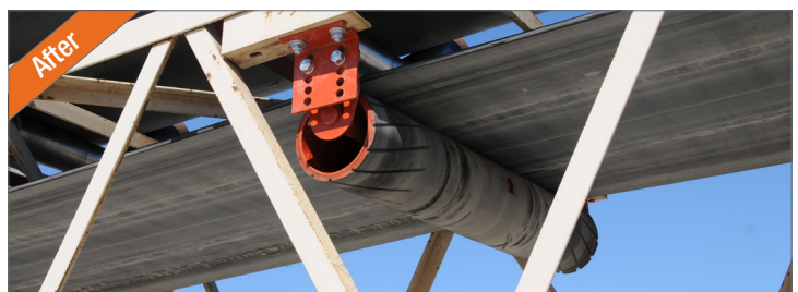
Belt Straightened Immediately After Installation
