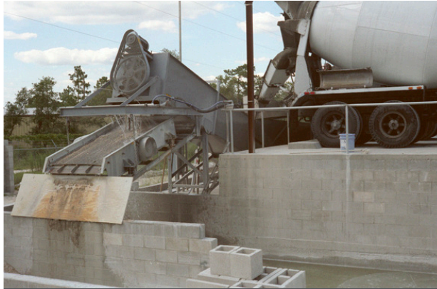
UNLOAD TWO READY-MIX TRUCKS AT ONCE
