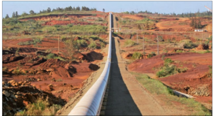
Conveyor Belt Covers
