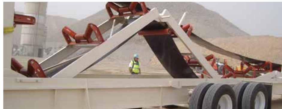
AN EXPERIENCED CREW CAN ASSEMBLE IN HOURS
