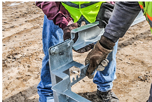
CHANNEL SECTION CONNECTING TO STAND
