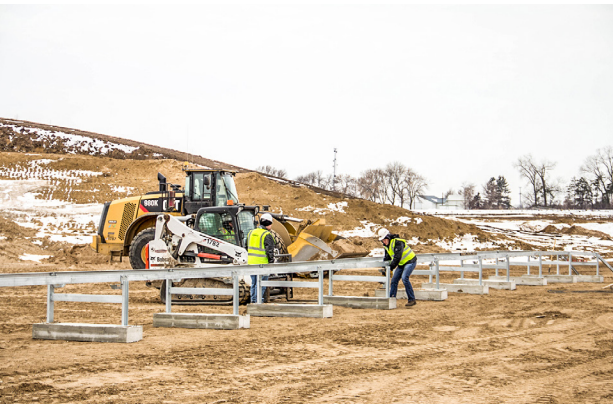
SECTIONS SPAN 10-FEET
